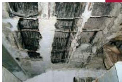
Fig. 8 Detail of concrete with cavities of the column of the Large Hall in the place of boring
