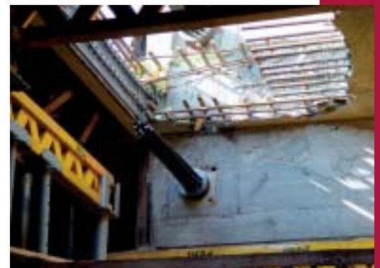
Fig. 6 Temporary breakout for the stressing jack
