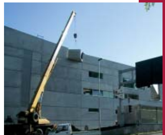
Fig. 6 Protruding facade from large-size prefabricated reinforced concrete panels
