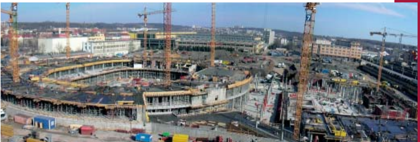
Fig. 10 View of the building under construction
