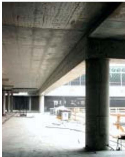
Fig. 9 Transient structure above the supply yard – span 22 m
