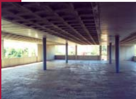
Fig. 16 Ceiling panels from visual concrete with a panel band
