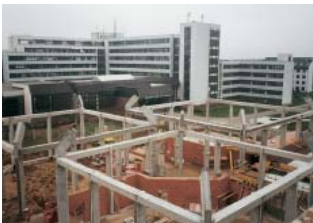
Fig. 17 Columns with peripheral collars
