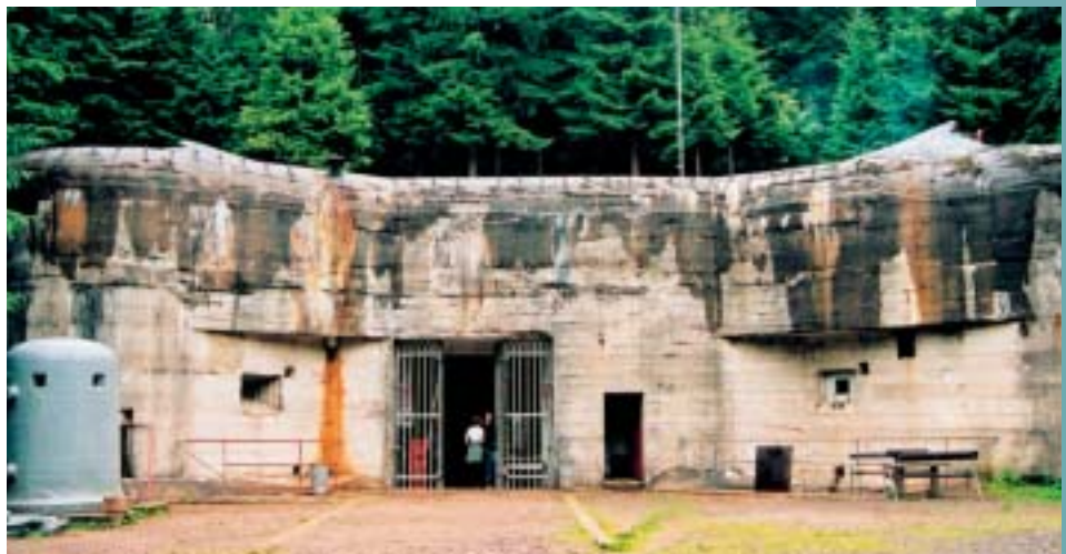
Fig. 6 The entrance to the "Bouda" fortress – contemporary situation
