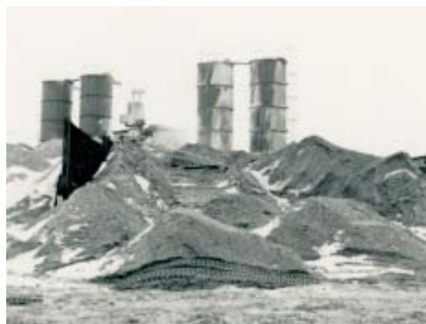
Obr. 13 Skládka kameniva u výroby transportbetonu z počátku 70. let Fig. 13 Dump aggregate at the mixing plant at first 70. years
