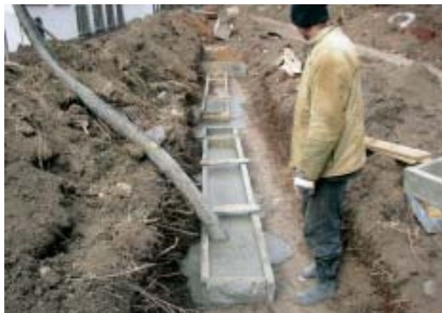
Fig. 6 Reconstruction of sewerage in Brno – filling of the formwork
