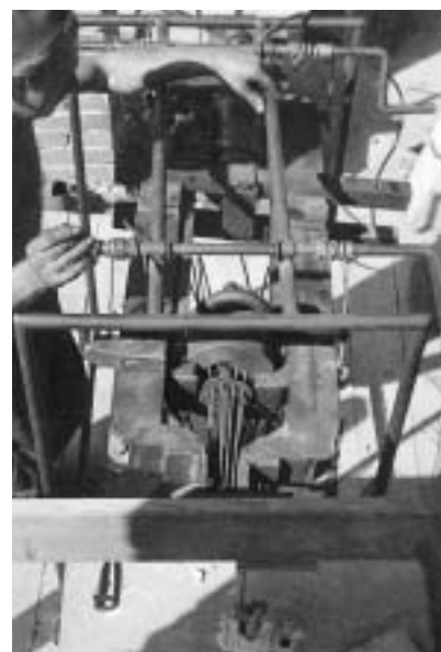
Obr. 2 Kleště Baraba Fig. 2 Prestressing equipment Baraba
