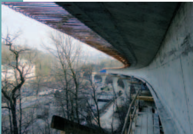
Fig. 1 Hlubočepy viaduct – general overview
