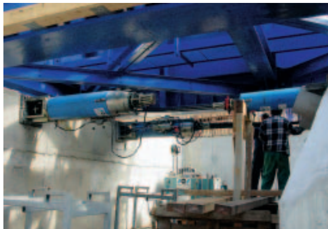
Fig. 2 Launching equipment installation, synchronized pulling and retaining strand jacks
