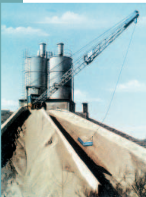
Obr. 8 Betonárna Elba Obr. 8 Concrete mixing plant Elba
