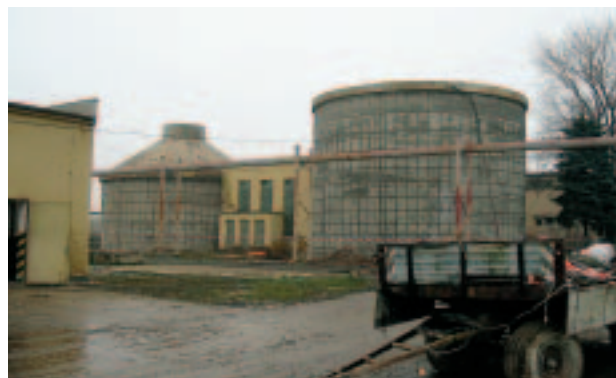
Obr. 2 Pohled na nádrže v ČOV Kralupy Fig. 2 View of the tanks in WWTP Kralupy
