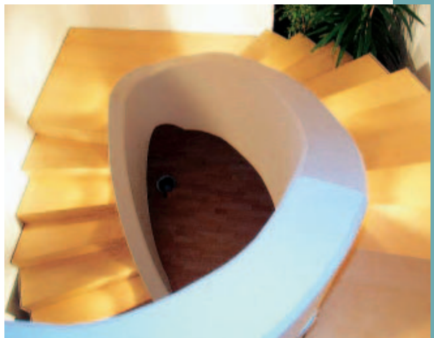
Fig. 7 View of the staircase from the top landing
