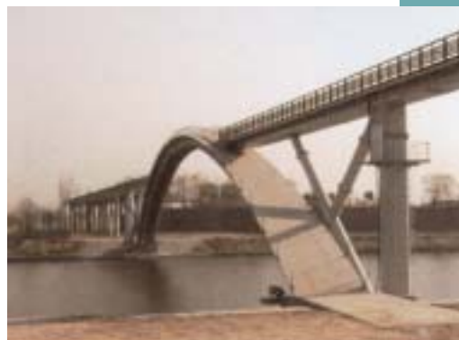
Fig. 4 Seoul Peace footbridge, the span length of the arch 120 m, in the 60m central part with the pedestrian traffic directly on the arch
