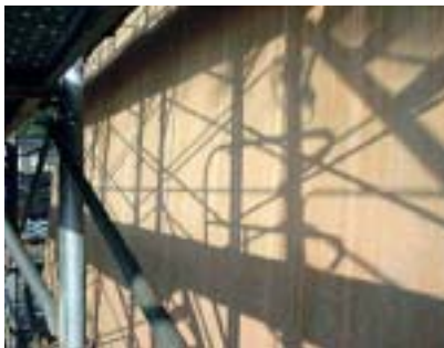
Obr. 7 Pohled na povrch mostu Fig. 7 View of the bridge surface
