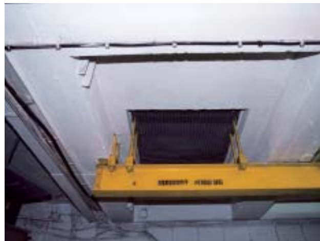
Fig. 5 The same space after packing repair with fire-protection coating
