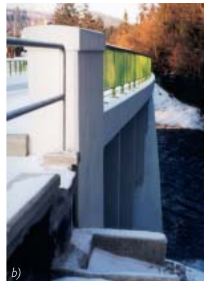
Fig. 6a), b) Completed repair of the bridge arch, cornices and the new railing
