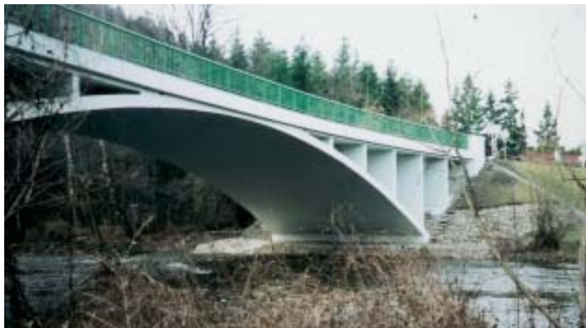
Fig. 7 Repair and new improvement of the banks below the bridge
