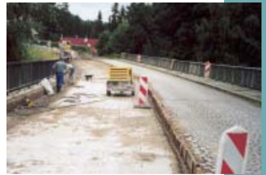
Fig. 4 Repair of a part of the bridge while maintaining operation in its other part
