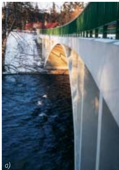
Fig. 6a), b) Completed repair of the bridge arch, cornices and the new railing
