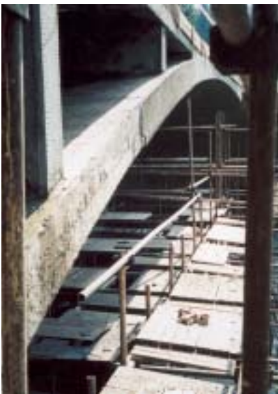
Fig. 5 Cleaning the bridge arch from degraded concrete
