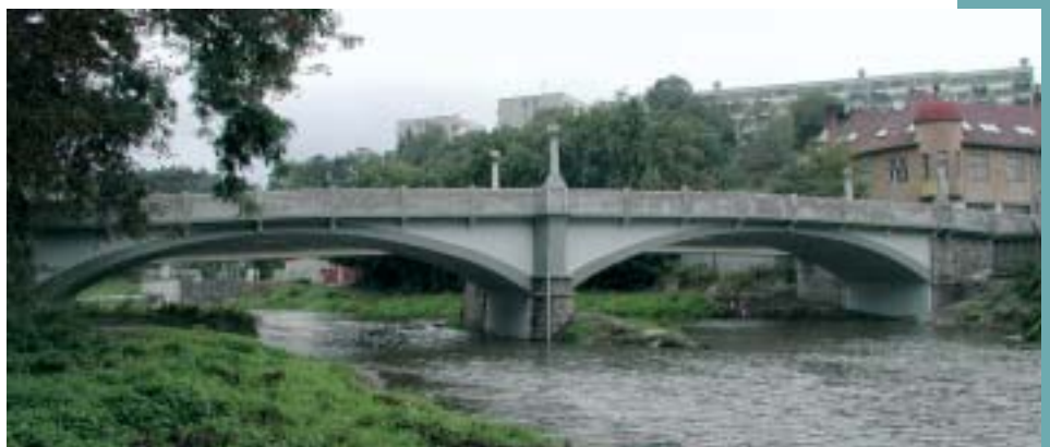
Obr. 7 Most po opravě – celek Fig. 7 Bridge after the overhaul – general view
