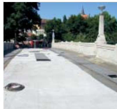
Fig. 3 Applying insulation
