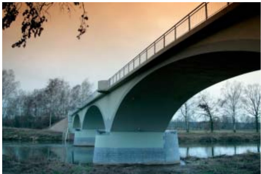
Fig. 11 General view of the bridge after the reconstruction completion
