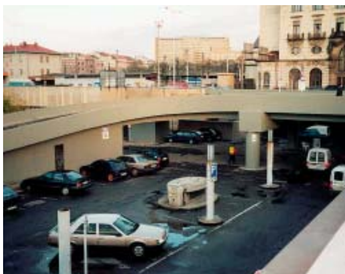
Obr. 2 Hlavní nádraží v Praze – Parking Wilsonova, rekonstrukce a sanace Fig. 2 Main Railway Station in Prague – Parking in Wilsonova Street, completed reconstruction and rehabilitation
