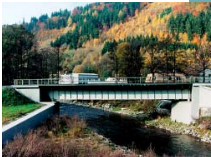
Obr. 2 Železniční most u Hanušovic po rekonstrukci Fig. 2 Railway bridge near Hanušovice after reconstruction
