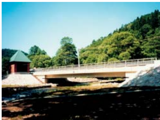
Obr. 4 Pohled na nově postavený most u obce Vlaské Fig. 4 View of the newly built bridge near Vlaské village
