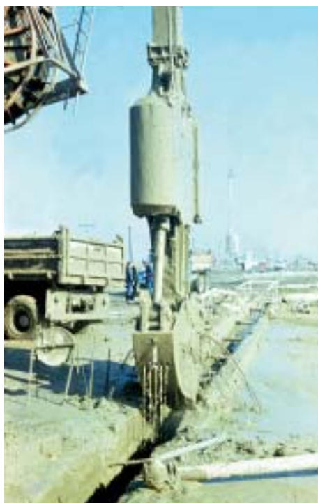
Fig. 5 Cement-bentonite suspension in the diaphragm wall
