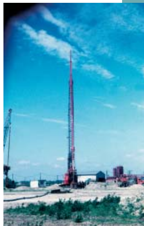
Fig. 6 The excavating equipment for diaphragm walls
