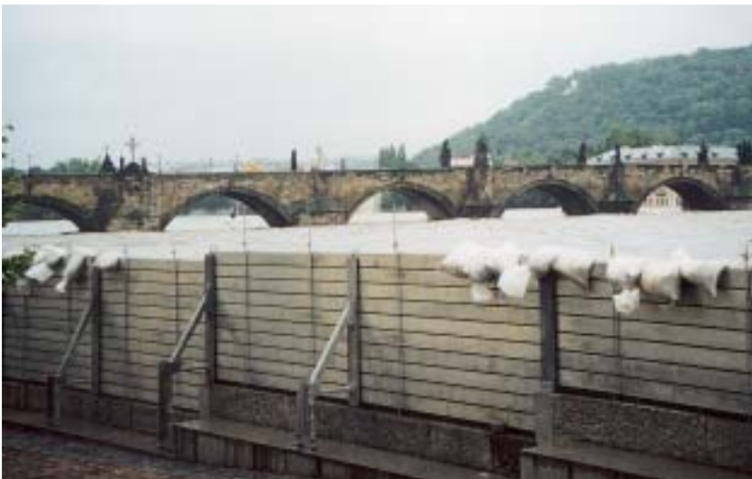
Fig. 5 View of Charles Bridge over the mobile flood defence during the flood in August 2002
