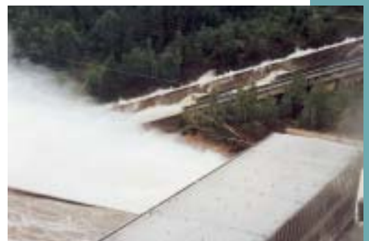
Fig. 5 Hydraulic structure Orlik; unplanned water outflow through flumes of ship-lifts at the time of the flood culmination
