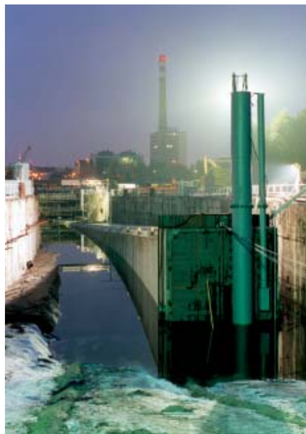
Fig. 3 Metro tunnels under the Vltava River
