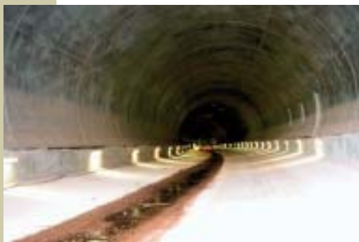
Obr. 5 Pohled na hotový tunel Fig. 5 View of the completed tunnel
