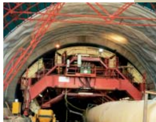
Fig. 3 Preparation works before concreting of the secondary jamb of the tunnel
