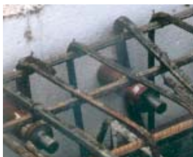
Fig. 7 Shear load connectors CRET 203 Entertainment Centre Černý most
