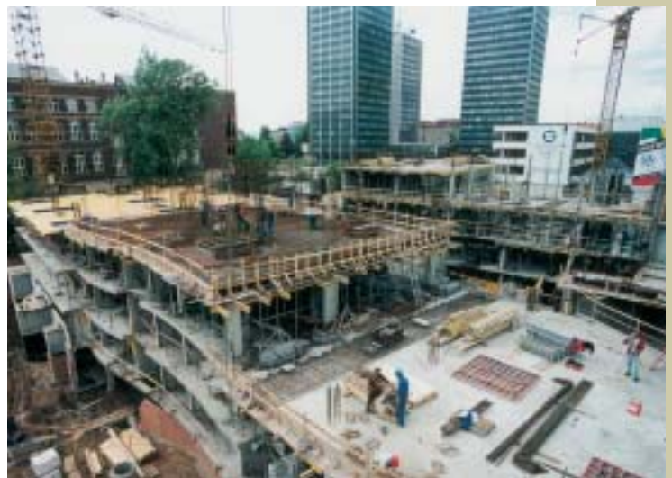
Fig. 6 The 3 rd above-ground storey of the South wing – floor slab
