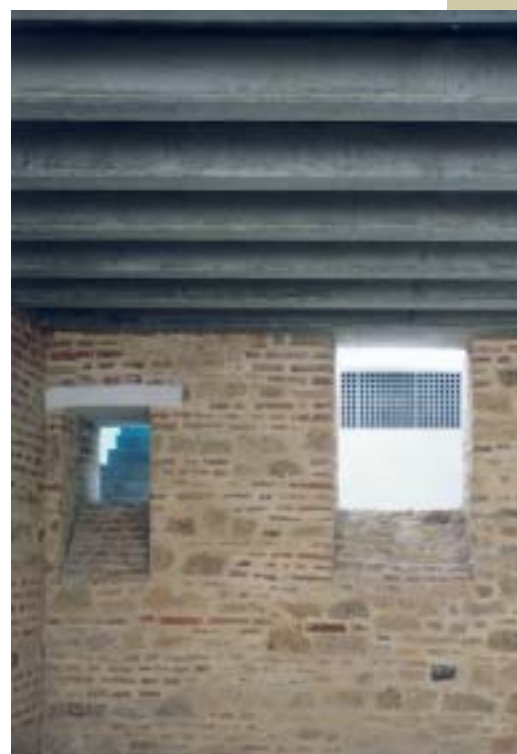
Fig. 6 Basement of the Palace with unplastered monolithic concrete floors
