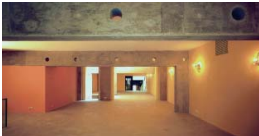
Fig. 5 Space inside the shop in Palace Langhans with unplastered reinforced concrete girders and trowel-applied floors
