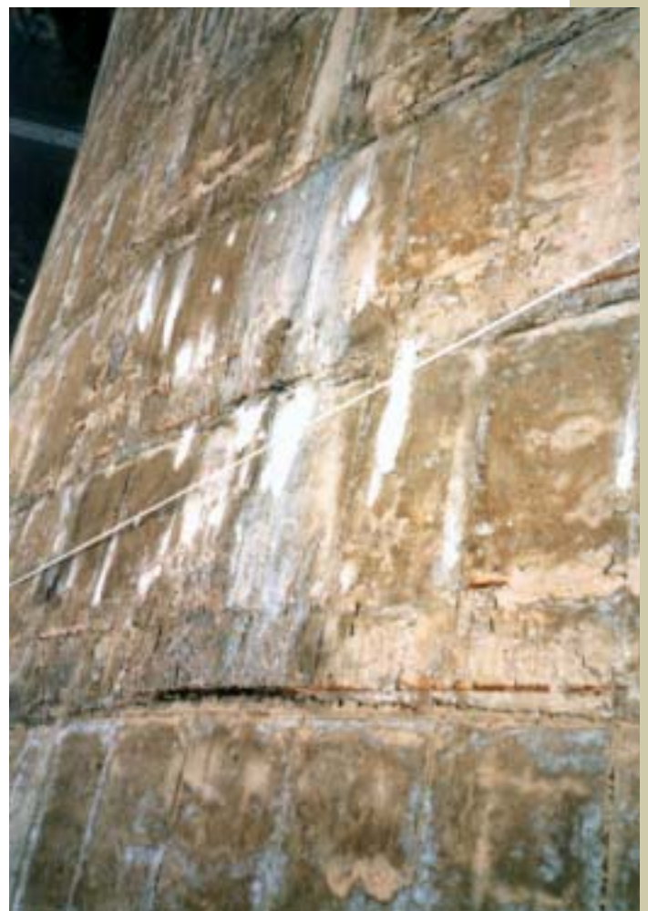
Fig. 1 View of the heavy pitted surface of the cooling tower cladding
