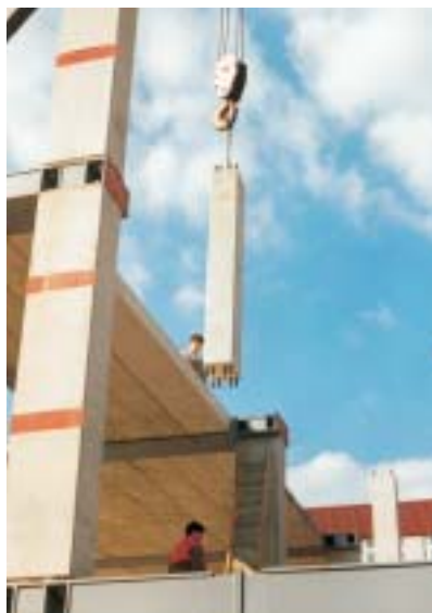
Fig. 6 Assembling of building of Screen house, Praha-Malešice
