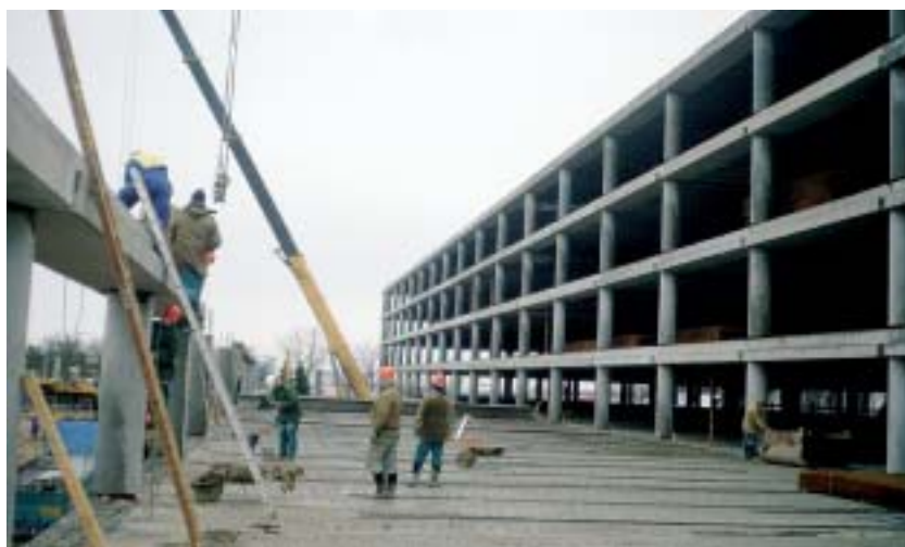
Fig. 8 Step-by-step assembly performed by sections
