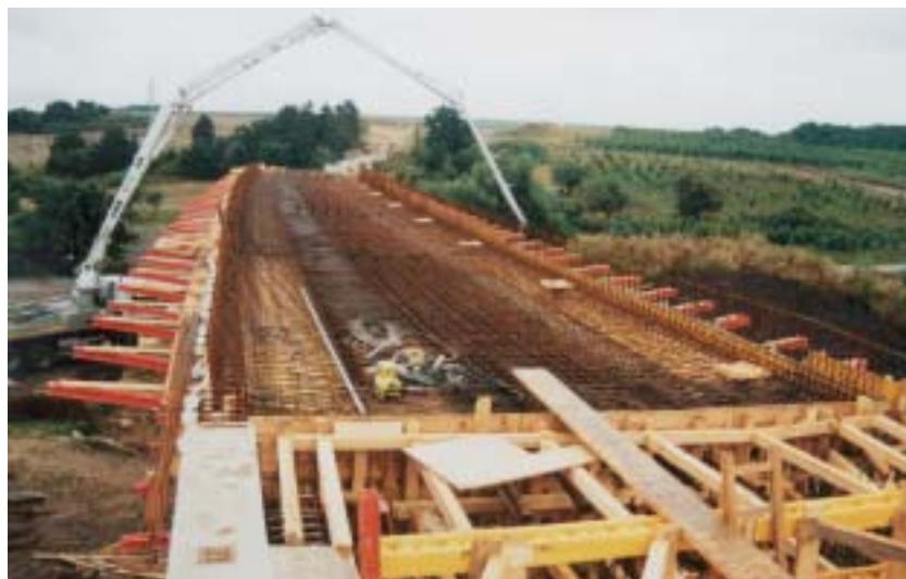
Fig. 1 View of the first concreted section – 315 m 3 concrete volume
