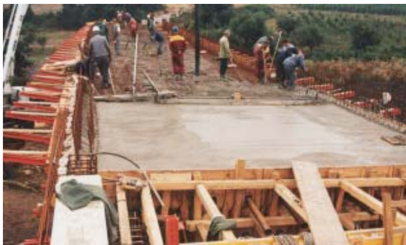
Fig. 4 Process of concreting of the centering
