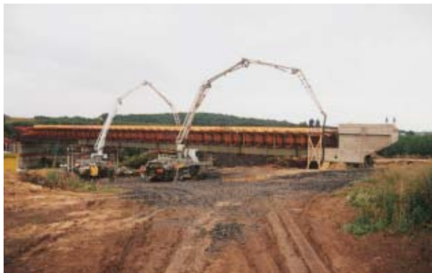
Fig. 2 Placement of pumps throughout the concreting period
