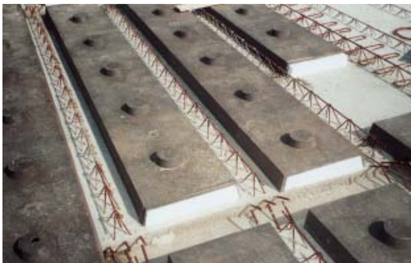
Fig. 4 Assemblage of installation shell fillers
