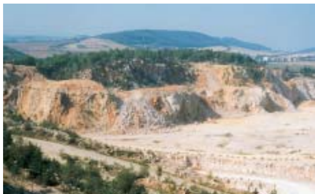
Fig. 3 Morphology of the same area during finalization works
