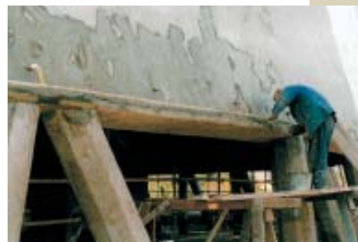
Fig. 3 Completed reprofiling of the PCC jacket using SAN-B mortars
