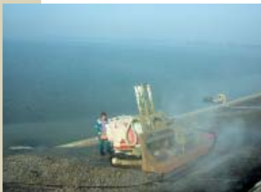
Fig. 3 Works on Goczalkowice dam
