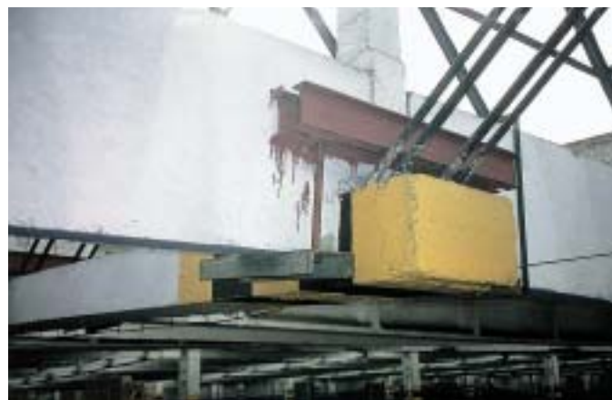
Fig. 5 Additional and yet low-quality fitting of rafters on prestressed ground plate of the joining beam
