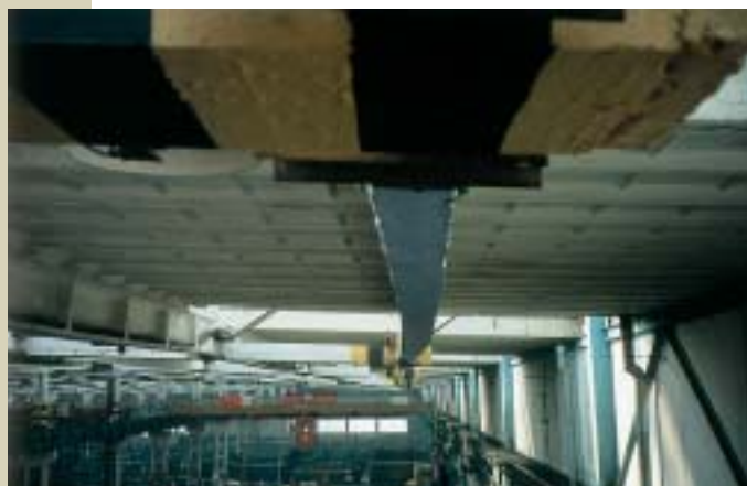
Fig. 4 View of the bottom of the roof. Evident sag of U-type rafter
