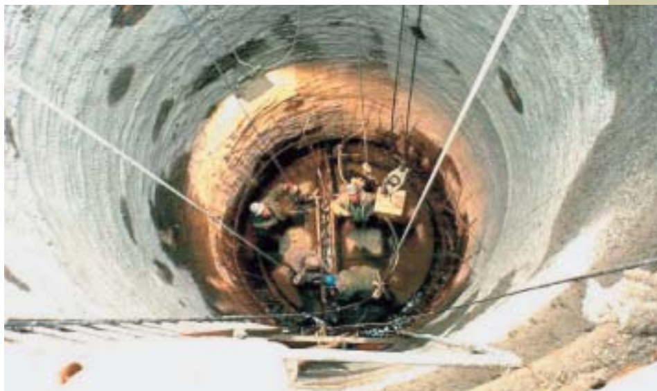
Fig. 2 Concreting of the secondary lining
