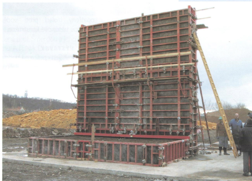
Fig. 1 Formwork of the model for experimental verification of the casting sequence
