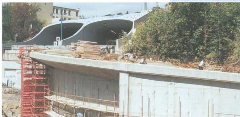
Elevated approach to Strahov tunnel
