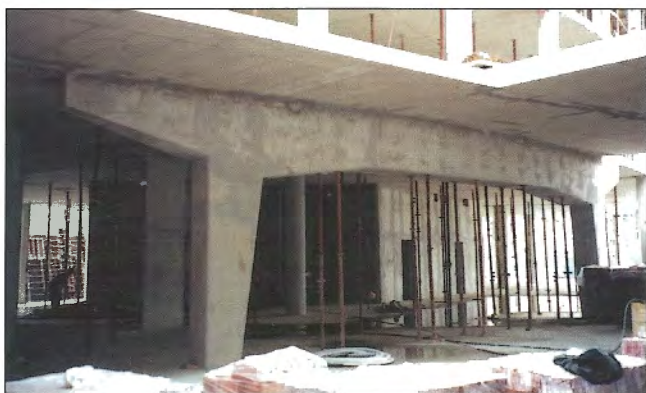
Obr. 12, 13 – Objekt K - rám ve vstupní hale / Building K - frame in the entrance hall
