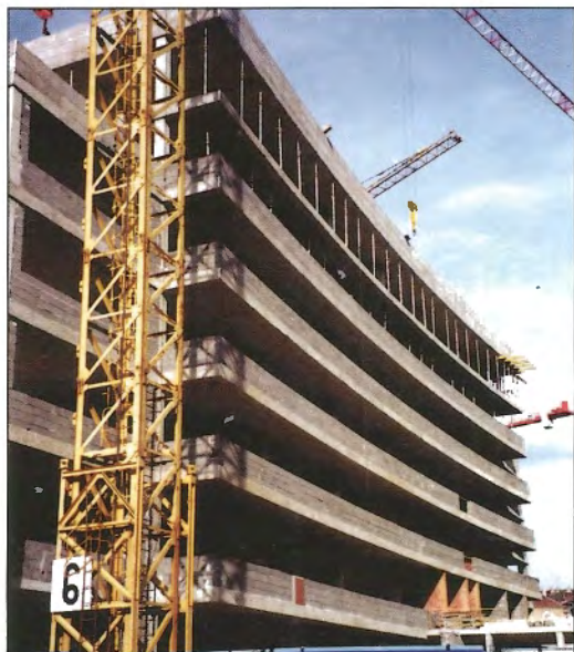
Obr. 16 – Objekt JV - pohled / Building JV - view
