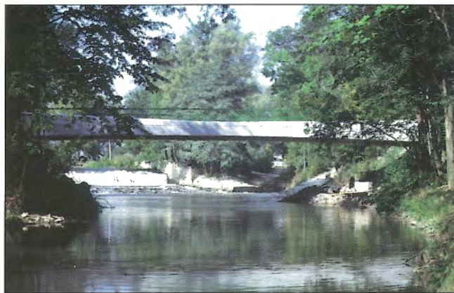
Obr. 9 – Most v Jaselské – Pohled k jezu / Bridge at Jaselská – View of bridge and weir
