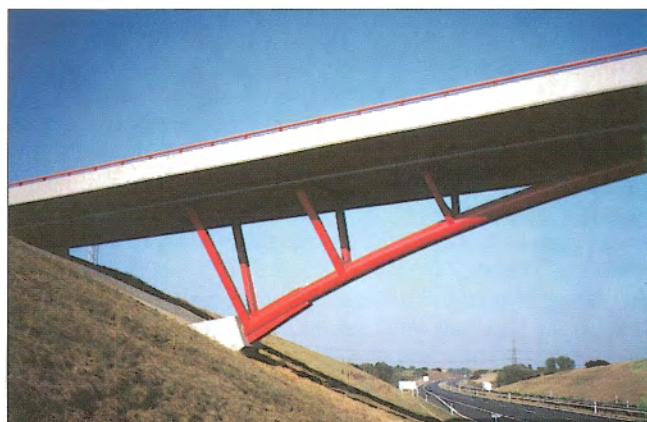
Obr. 10 – Oblouk a mostovka / Arch and deck
