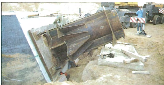
Obr. 18 – Pata oblouku / Arch spring
