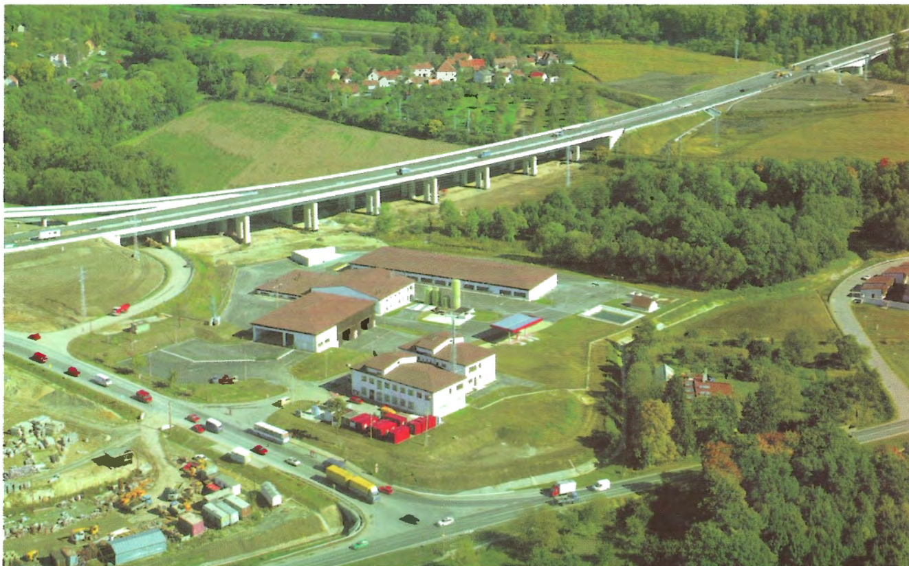
Obr. 1 - Letecký pohled na most / Aerial view of the bridge
