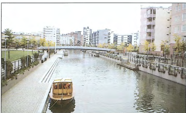
Obr. 3 – Kanál protínající sídliště Ruoholahti / Water channel going through the Ruoholahti housing estate
