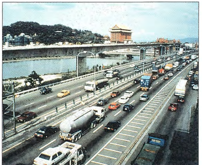
Obr. 22 – Pohled na most / View of the bridge
