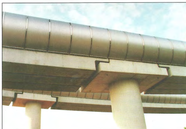
Obr. 2 – Viadukt KW 1643, detail / Viaduct KW 1643, detail
