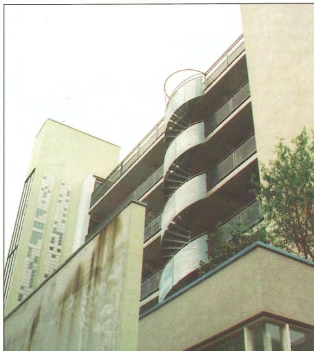
Obr. 5 – Jiná budova nemocnice / Another hospital building
