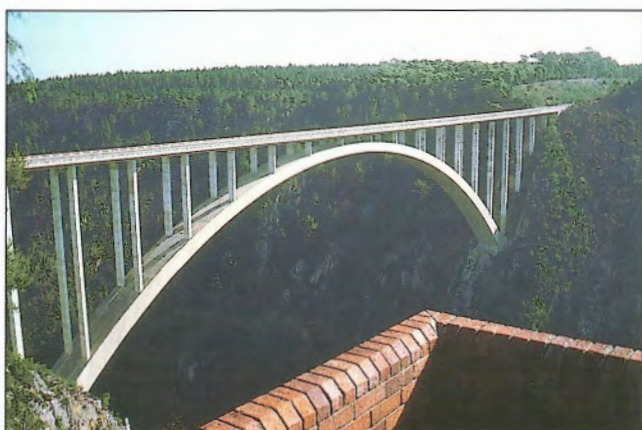
Obr. 4 – Most Bloukrans /Bloukrans Bridge
