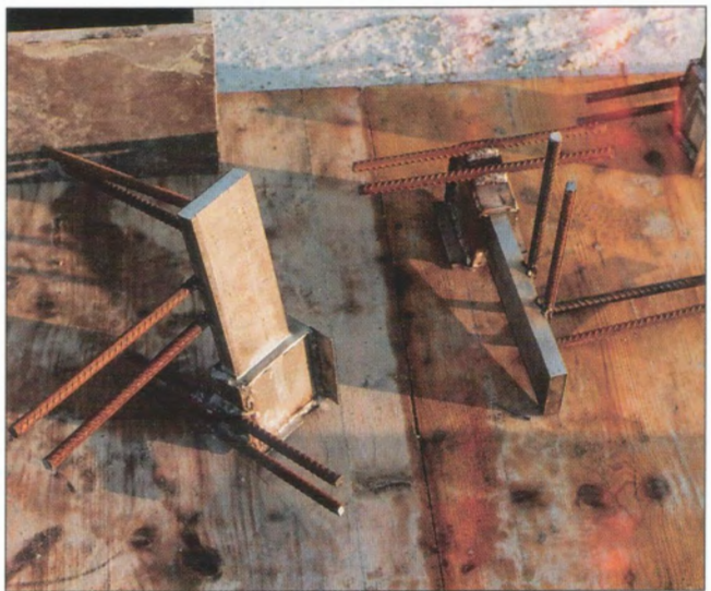
Obr. 5 – Posuvné klouby v pouzdrech / Sliding joints in sheaths
